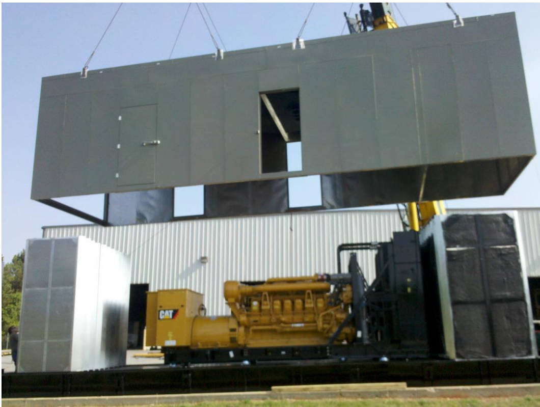
70 dB(A) @ 1 mtr enclosure on a 2000 kWe gen set on a UL142 3000 gallon tank.
