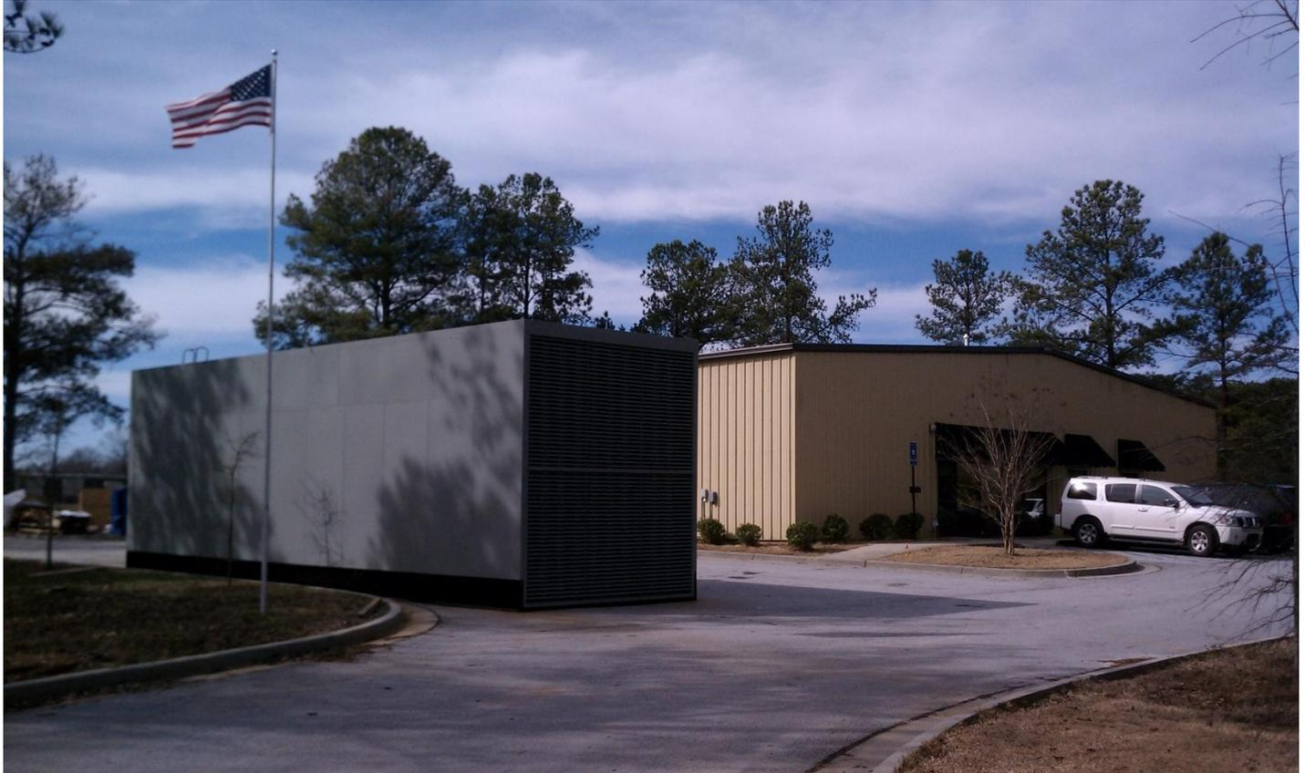
In this photo is the first 3000kWe genset to be delivered in the state of Georgia! It is 43' long x 12' wide and nearly 14' tall. Our scope called for an attenuation level of <math><86\text{ dB(A)}</math> at 1 meter. The 8 hour witness test proved we had not only met that, but beat it! With the noisiest side (just under the exhaust side outlet) reading 84 dB(A) at 1m and the side shown reading 73 dB(A) at 1m!
