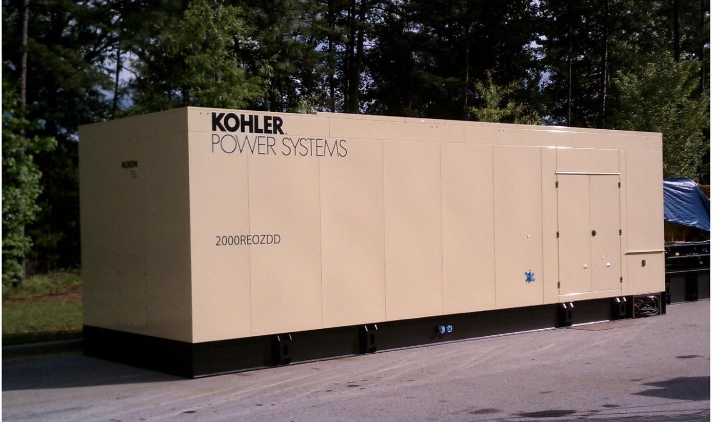
In this photo is a 2000kWe genset which was delivered in Georgia. It is 411" long x 12' wide and 12' tall. Our scope called for a Walk-in Enclosure, an attenuation level of <math><83\text{ dB(A)}</math> at 7 meter, and the installation of a 3000A circuit breaker with an external custom buss bar cabinet. The cables were run in a custom tray below the floor. Fuel supply and return piping was also under the floor, within the skid base. All to ensure a safe, neat work area within the enclosure!
